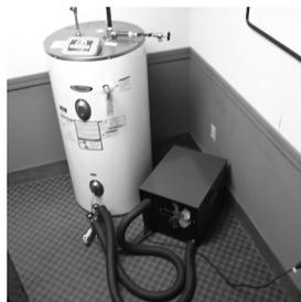
Once all hoses are connected, and the hoses are properly insulated, the plumbing portion of the installation is done.
