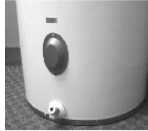
Locate drain valve at bottom of tank.
