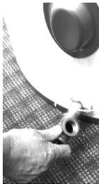
Next, insert one of the two brass "T" fittings, (item 103) onto the exposed end of the nipple, and tighten snugly. Leave the open "T" approximately in the vertical position.
