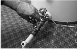
Now, apply thread seal tape to, and install the second valve, (item 104), onto the second "T" fitting.
