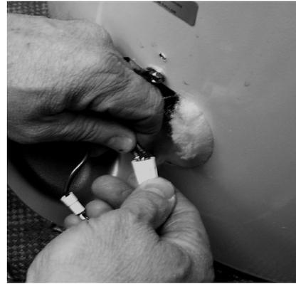
Wire tie the bare lead from the Geyser to the lead just removed from the tank, using the wire nut that comes with the Geyser. Electrical tape must be used to seal this connection. Take the second wire from the Geyser (the one with the terminal connector) and connect it to the terminal where you just removed the lead from the tank.
